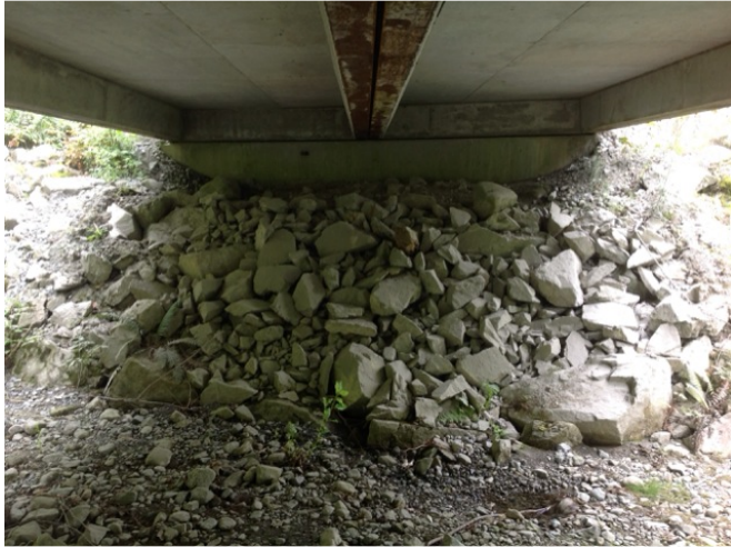
Left Bank Abutment when facing downstream
