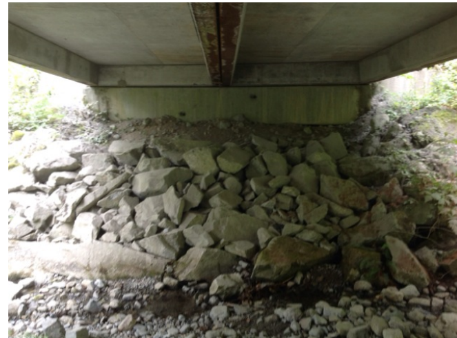
Right Bank Abutment when facing downstream
